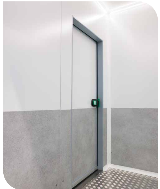
PVC interior coating
